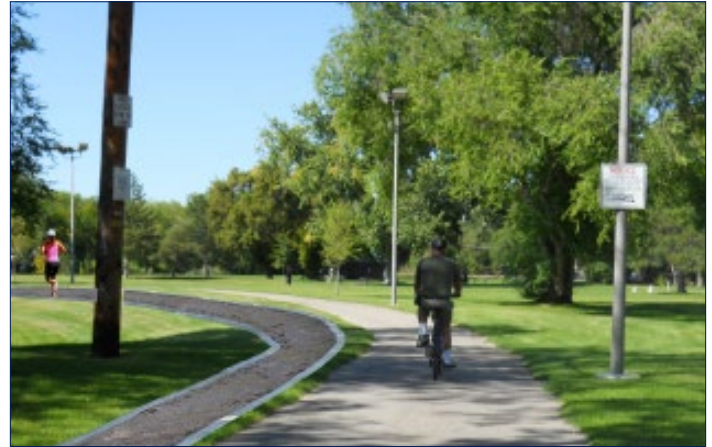
An additional trail, where spaces allows, can prevent conflicts between different users on the Jordan River Parkway and create a safer space for all users.
