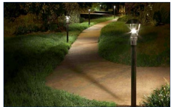
Bollard lighting that minimizes the light directed outside of the trail corridor.
